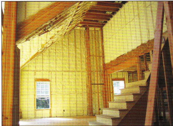
OPEN-CELL SPRAY-FOAM NEW CONSTRUCTION
