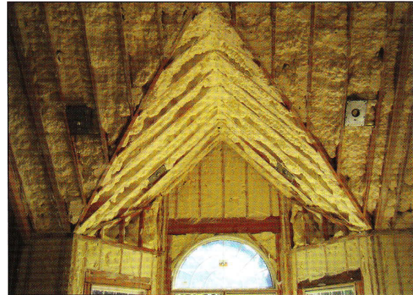
OPEN-CELL SPRAY-FOAM NEW CONSTRUCTION
