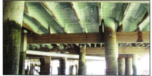
The underside of deck over the water winterized with a glass enclosure and radiant floor heat
