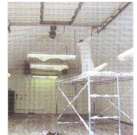
Highway Department Truck Repair Shop - needed a Fire Rated Thermal Insulation
